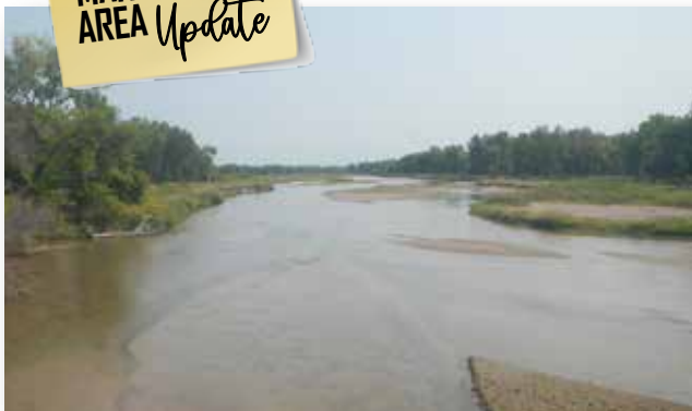
Platte River at Darr Bridge has been cleared of phragmites that severely restricted the water flow in past years. Herbicides were applied by helicopter and by airboat.
