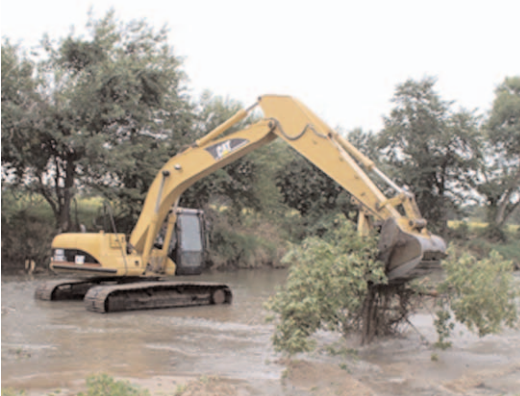
River channel cleanout on the Little Blue River being performed by Frahm Construction.
