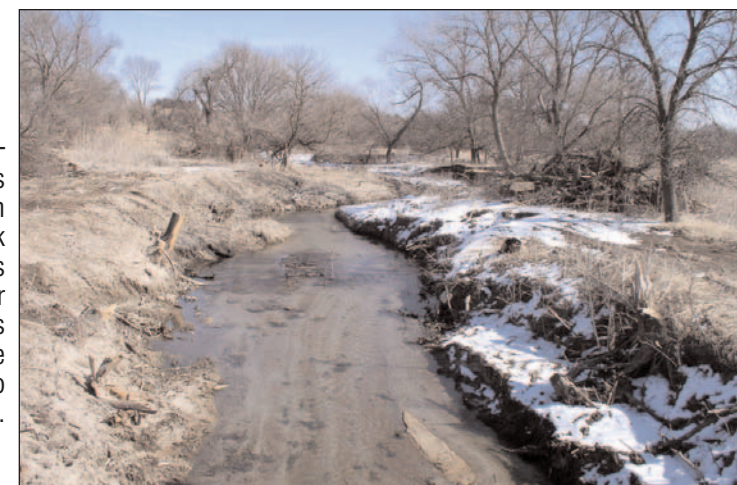
After – Water flows unobstructed in Turkey Creek after work was done to clear channel debris and remove trees close to the creek bank.
